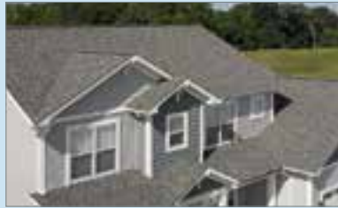
Roofing and Ventilation
