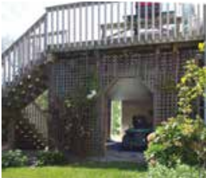
Under the deck is a perfect area for storage of frequently used outdoor toys, lawn and garden equipment and more.
